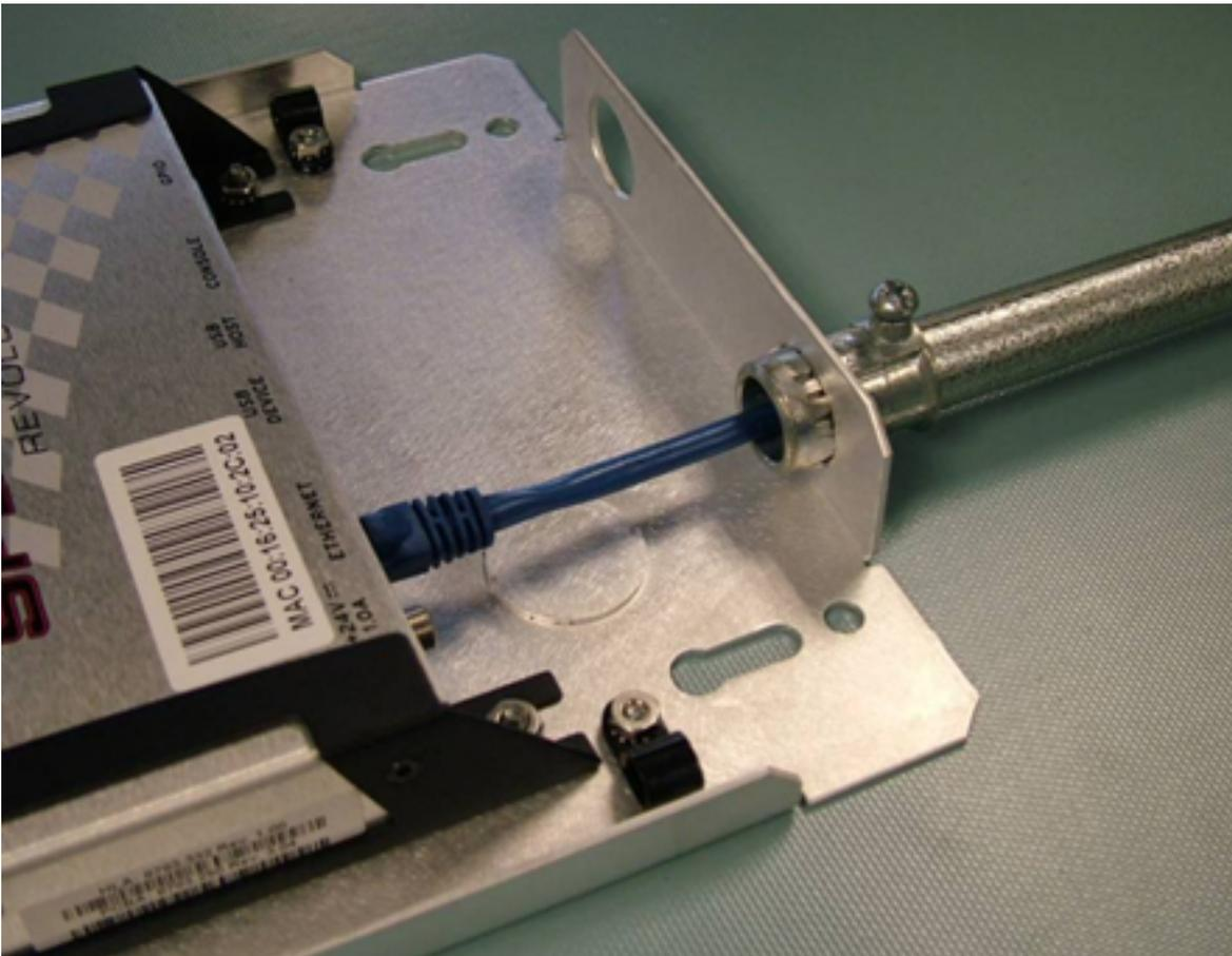
**Figure C.5 ½ inch conduit with a snap in flange connector**
